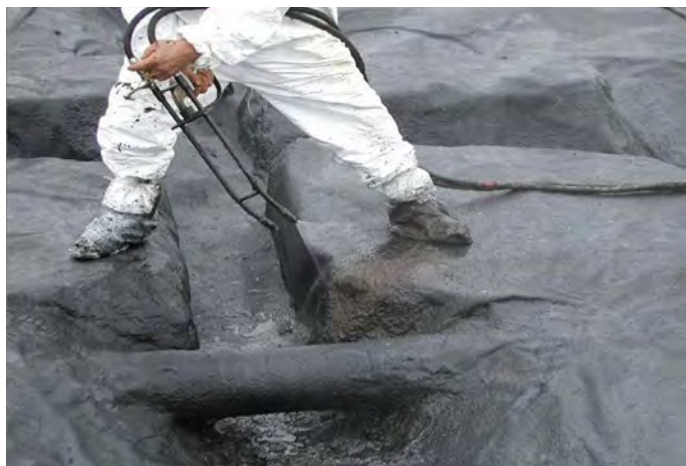
Figure 3.4-J Spraying Over Leakage Point
