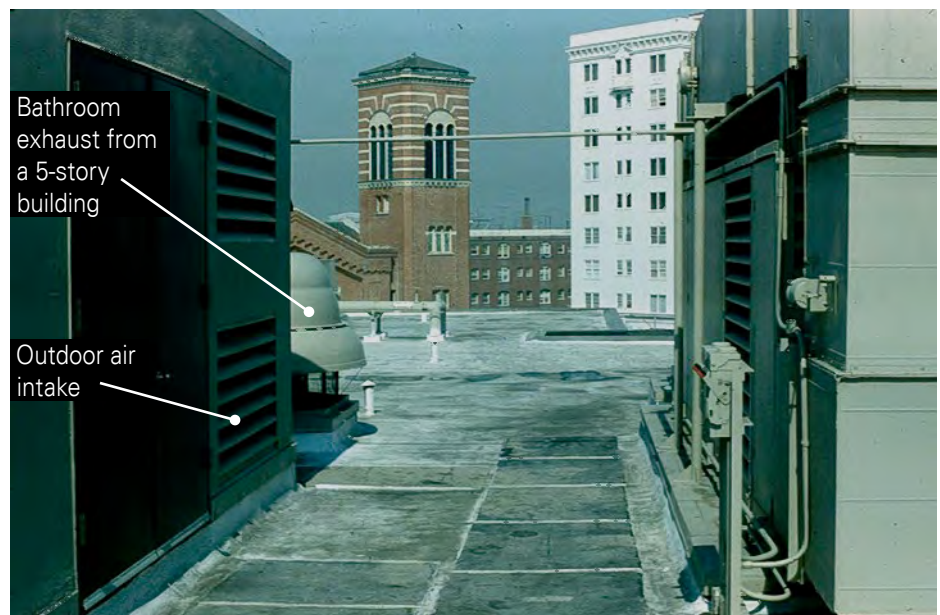
Figure 3.2-B HVAC Outdoor Air Intake Located Downwind of and in Close Proximity to Main Bathroom Exhaust of a Five-Story Office Building Photograph courtesy of Hal Levin.
