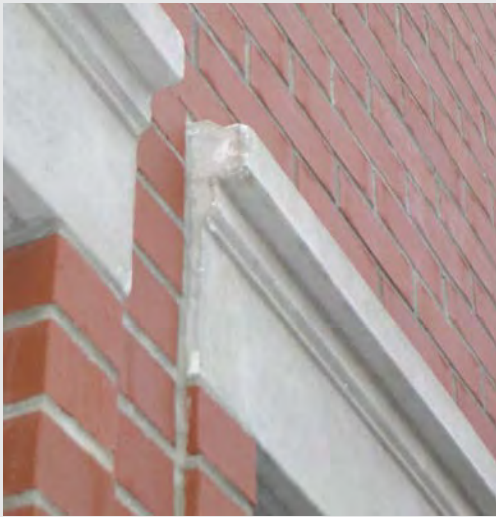
Figure 3.6-L Lintels Designed to Make it Uncomfortable for Pigeons to Roost Photograph courtesy of Terry Brennan.
