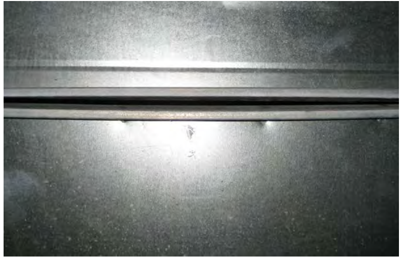
Figure 6.3-C Example of Excessive Duct Leakage Due to Improper Installation/Sealing Photograph courtesy of Jim Hall.
