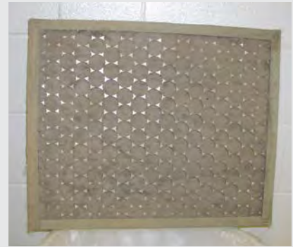
Figure 1.5-F Long-Unchanged Outdoor Air Filter that Became Clogged and was Sucked Out of the Filter Rack
