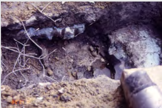
Figure 2.6-C Failure of a Three-Ply Asphalt/Felt Membrane beneath a Roof Garden Resulting in Root Penetration into the Roof Substructure Photograph copyright Justin Henshell.
