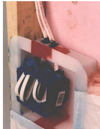
Figure 2.2-U Back Box that Fits around a Standard Electrical Box Photograph copyright Stephen K. Lentz.
