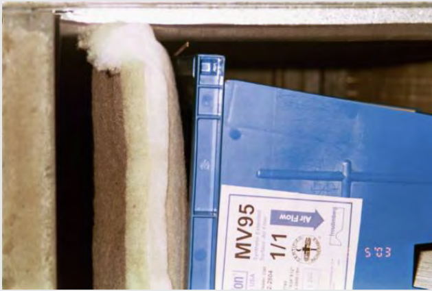
Figure 7.5-H Fallen Filter with Substantial Visible Gap
