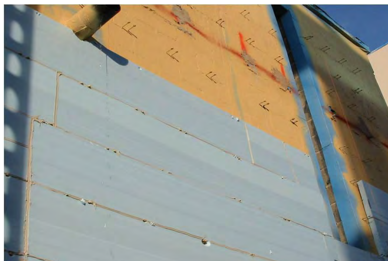
Figure 2.2-AC Well-Installed Rigid Insulation Embedded in Mastic with Sealed Joints
