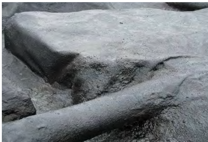
Figure 3.4-K Leak Eliminated—No Smoke Escaping
