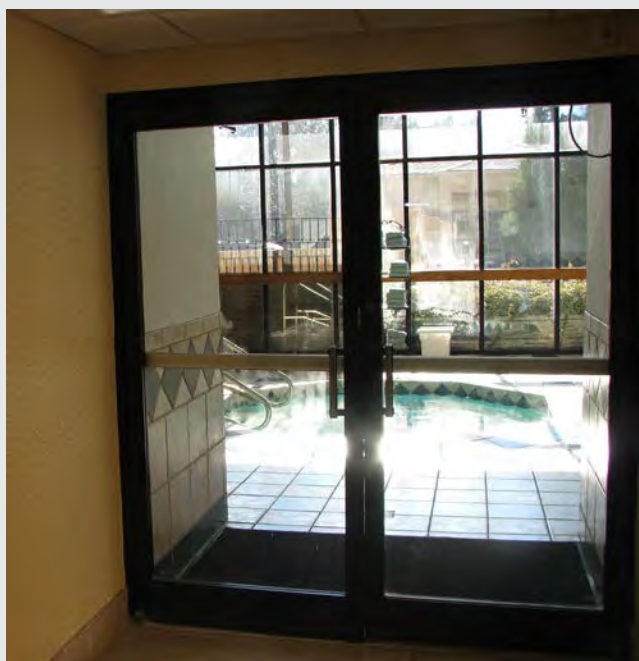
Figure 6.4-B Ill-Fitting Double Glass Doors
