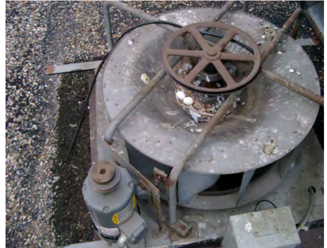
Figure 1.5-J Distributed Equipment on Roof—Packaged Roof Ventilator with Long-Broken Belt Photograph courtesy of Mark Hancock.
