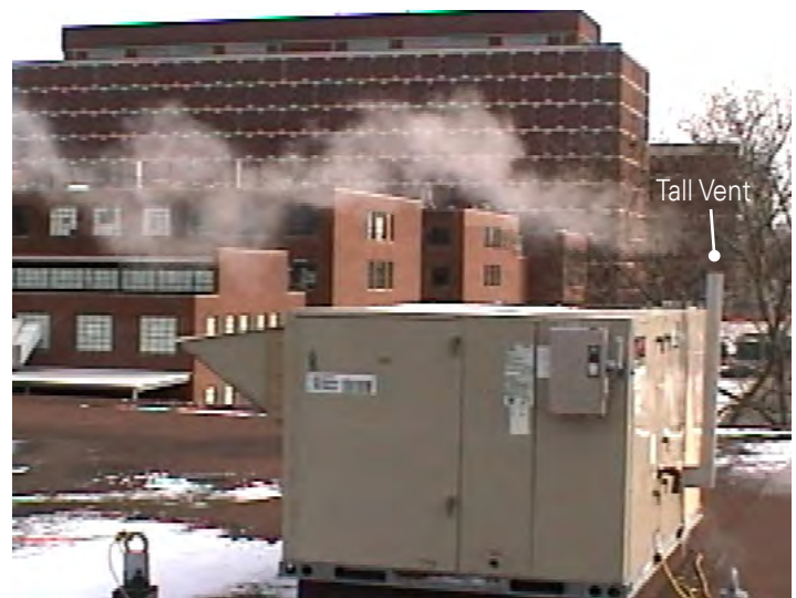
Figure 3.2-G Plume Dispersion from Tall Vertical Vent Photograph copyright Battelle Memorial Institute.
