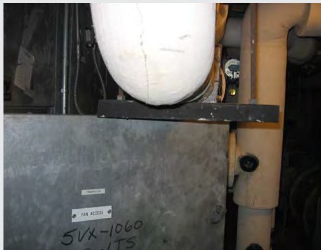
Figure 4.3-J Access Door Blockage
