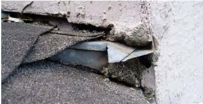
Figure 2.1-S Improper Roof Flashing Detail Photograph copyright Liberty Building Forensics Group®.
