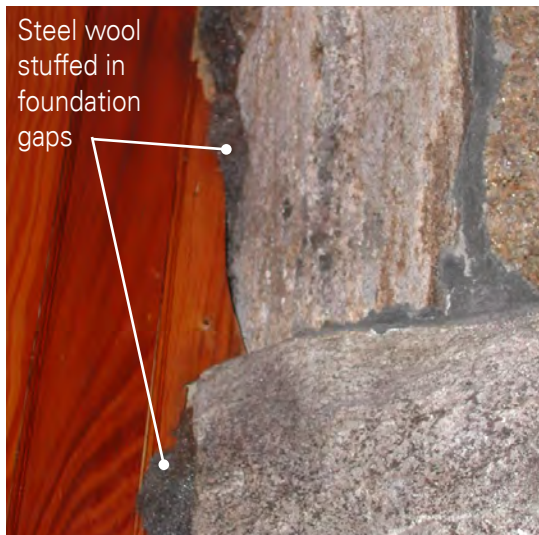
Figure 3.6-O Steel Wool Used to Block the Entry of Rodents Photograph courtesy of Terry Brennan
