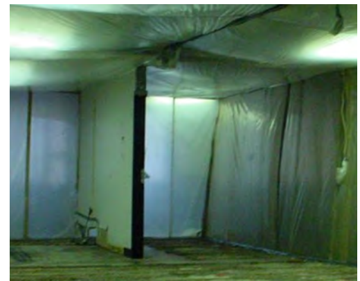
Figure 1.4-J Plastic Sheathing Isolating Construction Zone from Occupied Areas Photograph courtesy of Wayne Thomann.
