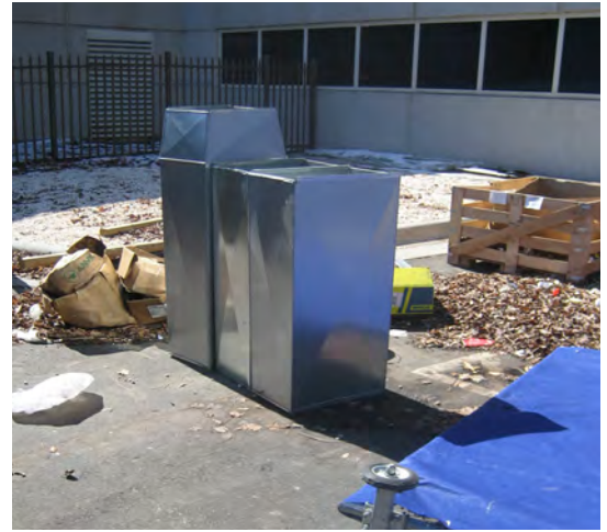
Figure 1.4-F Unprotected Storage of HVAC System Ducts at a Construction Site Photograph courtesy of Wayne Thomann.
