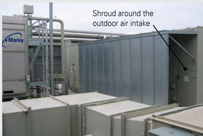
Figure 3.2-L Outdoor Air Intake Shroud Location Relative to Cooling Tower
