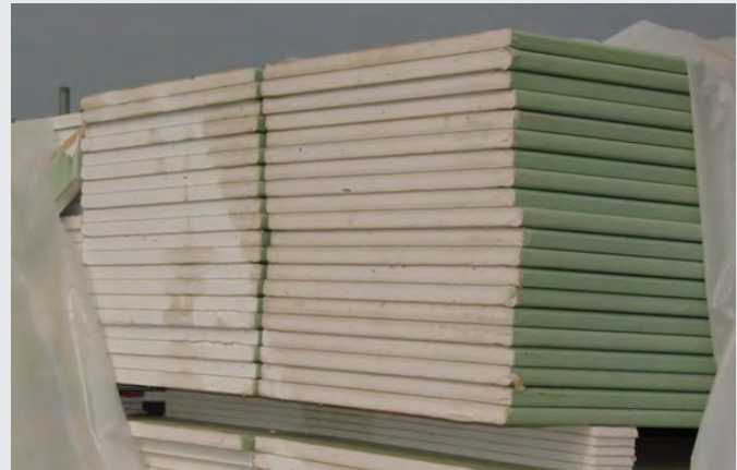
Figure 1.4-B Installation of Water-Sensitive Materials in an Exposed/Unprotected Structure
