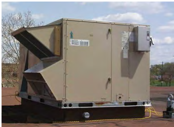
Figure 3.2-H Economizer Hood Installed on Packaged HVAC Test Unit Photograph copyright Battelle Memorial Institute.
