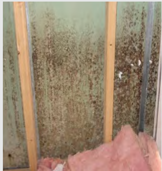
Figure 1.4-D Mold Growth from Wetting of Exposed Water-Sensitive Materials—Example 2
