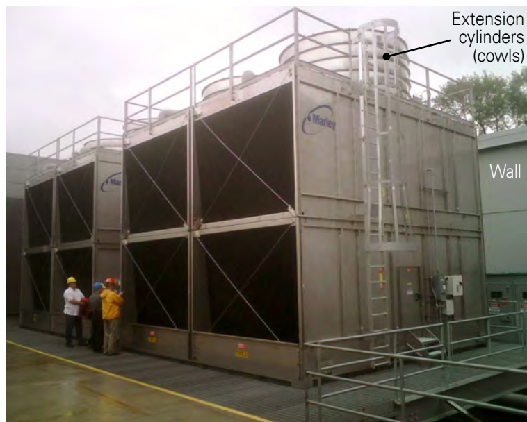
Figure 3.2-D Cooling Tower with Adequate Number of Extension Cylinders Added to the Exhaust Plume Photograph copyright SPX Cooling Technologies, Inc.
