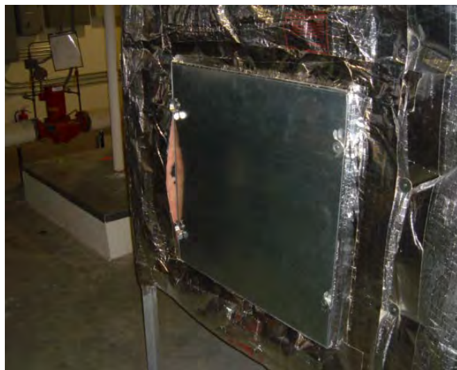
Figure 4.3-K Compromised Vapor Retarder at Access Door Installation Photograph courtesy of Wayne Thomann.
