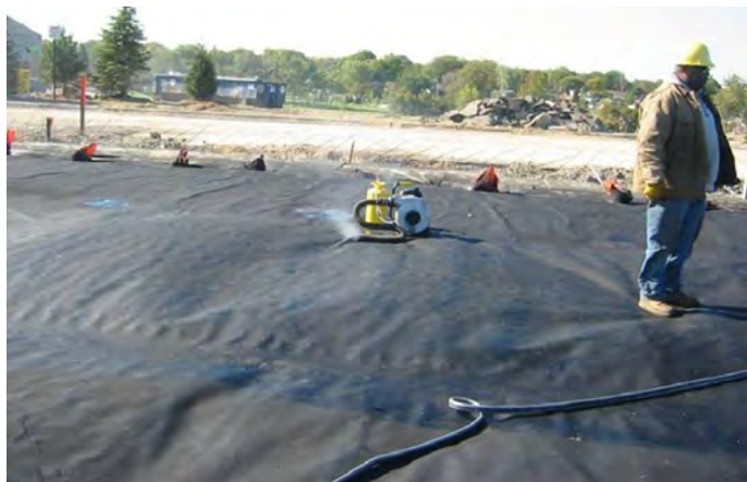
Figure 3.4-H Fan Injecting Smoke Under Membrane
