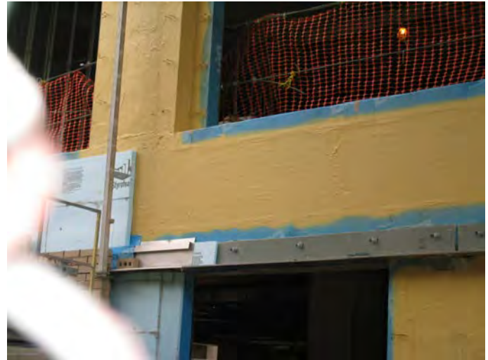
Figure 2.2-R Liquid-Applied Air Barrier Being Applied to Balance of Wall (Shepley Bulfinch Richardson and Abbott, Architect) Photograph courtesy of Wagdy Anis.
