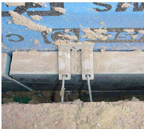
Figure 2.2-AB Poorly Installed Rigid Insulation in Brick Cavity with Air Gaps between and behind Boards
