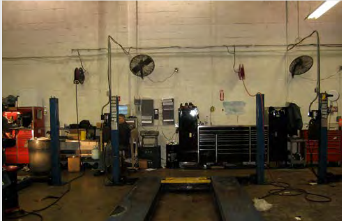
Figure 7.6-C Wall Fans in Vehicle Maintenance Shop Photograph courtesy of Larry Schoen.
