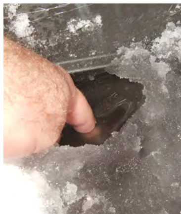
Figure 2.1-X Ice Dam Failure Close-Up Photograph copyright Liberty Building Forensics Group®.
