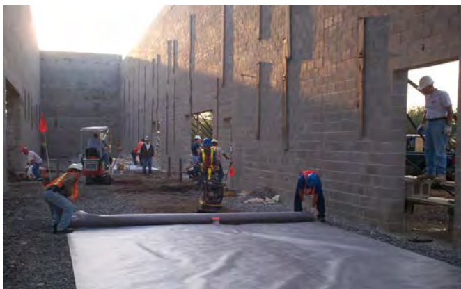
Figure 3.4-D Base Fabric (Non-Woven Geotextile) Installed to Protect Spray-Applied Gas Vapor Barrier Membrane from Underlying Aggregate, which Includes a Low-Profile Venting Network (see Figures 3.4-L and 3.4-M) Photograph copyright CETCO.
