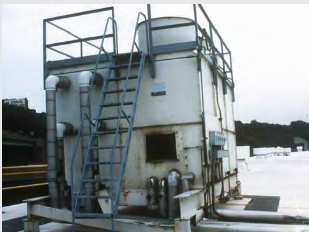
Figure 4.4-A Cooling Tower Found to be the Source of Legionnaires' Disease in Nearby Building
