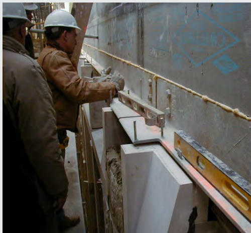
Figure 2.2-W Foam Sealant Applied between Insulation Boards
