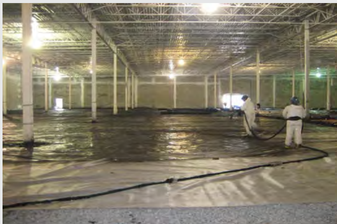
Figure 3.4-A Gas Vapor Barrier Being Sprayed onto Geotextile Base Fabric (Additional photographs from this project are shown in Figures 3.4-D, 3.4-E, and 3.4-G.)
