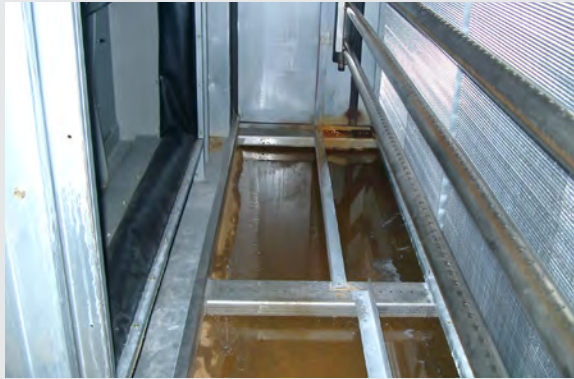
Figure 1.2-F Drain Pan with Standing Condensate Photograph courtesy of Martha Hewett.
