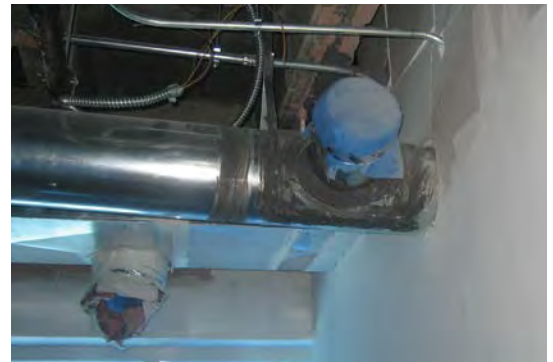
Figure 1.4-F Unprotected Storage of HVAC System Ducts at a Construction Site Photograph courtesy of Wayne Thomann.
