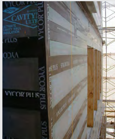
Figure 2.2-X Modified Asphalt Tape Photographs courtesy of Wagdy Anis.
