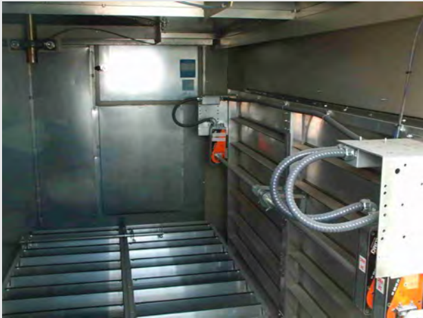
Figure 7.2-H Minimum Outdoor Air Dampers (to the Right) and Return Air Dampers (at the Bottom)
