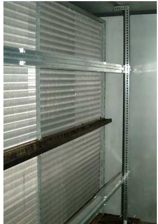
Figure 4.5-B Horizontal Lamp Placements for Coil Surface Disinfection Source: ASHRAE (2008), Figure 8.
