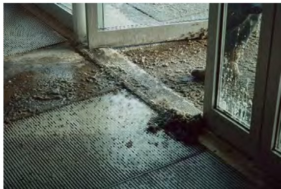
Figure 3.5-B Ineffective Track-Off System Photograph courtesy of Hal Levin.
