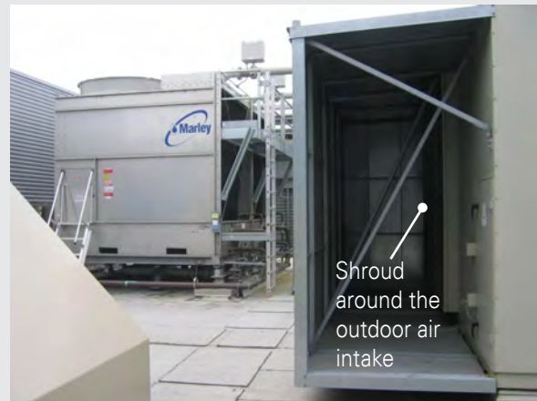
Figure 3.2-K Shroud Added to Outdoor Air Intake
