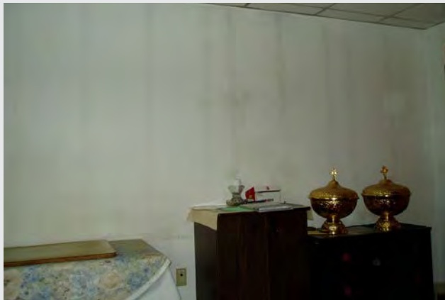
Figure 2.2-D Ghosting of Steel Studs on Walls Photograph copyright Wiss, Janney, Elstner and Associates, Inc.
