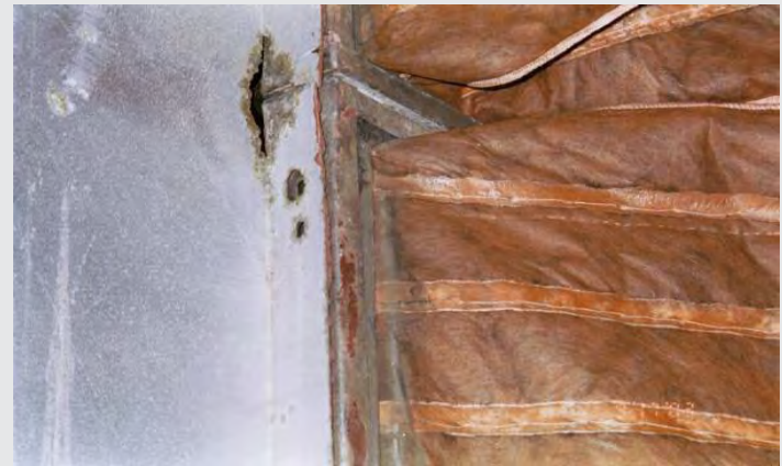
Figure 7.5-J Corrosion Penetration within an Air Handler
