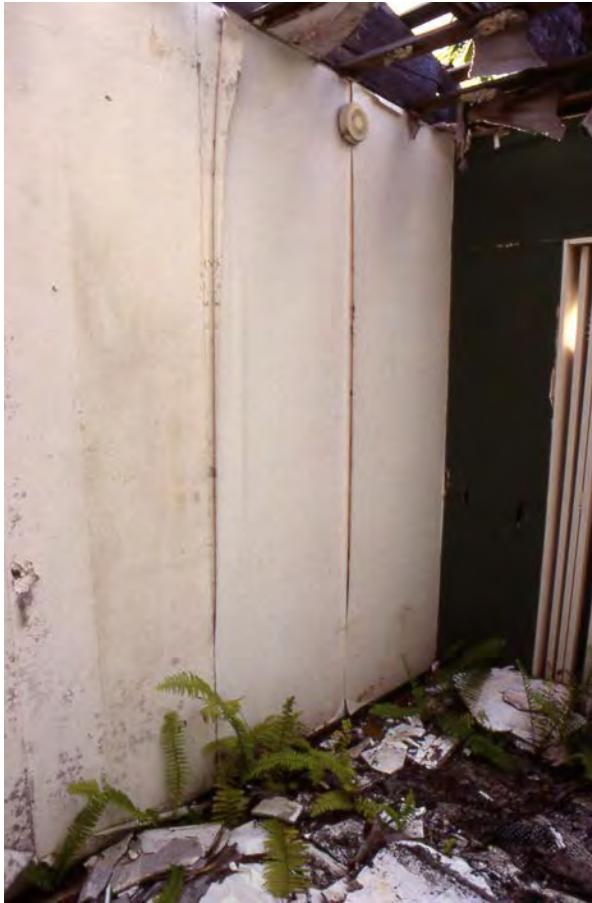
Figure 2.6-D Ferns Growing on the Flooring Indicating Conditions Moist Enough to Support the Growth of Fungi and Bacteria that Contribute to Building Biodeterioration Photograph courtesy of Phil Morey.
