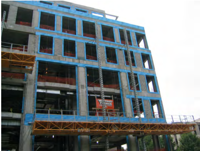
Figure 2.2-Q Peel-and-Stick Membrane Trimwork and Transitions Being Applied at Georgetown Law School (Shepley Bulfinch Richardson and Abbott, Architect) Photograph courtesy of Wagdy Anis.
