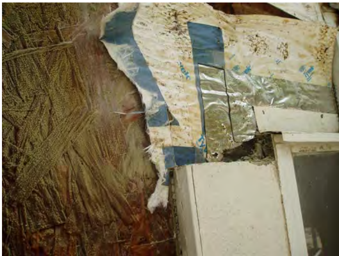
Figure 2.1-N Improper Window Flashing Photograph copyright Liberty Building Forensics Group®.
