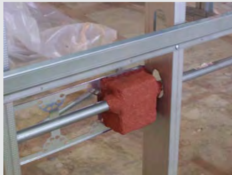
Figure 3.6-H Sealed Electrical Outlet in Common Wall between Apartments Photograph courtesy of Terry Brennan.
