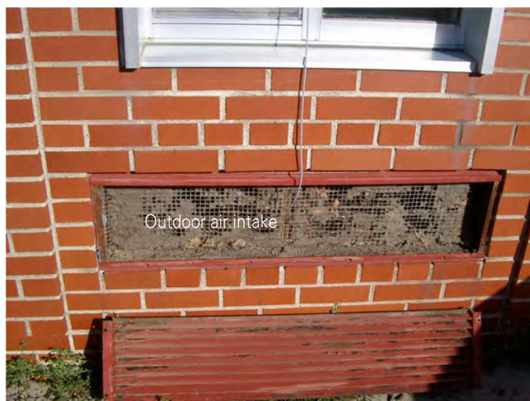
Figure 3.2-E Unit Ventilator Outdoor Air Intake Located Too Close to Ground Level Photograph courtesy of Mark Hancock.
