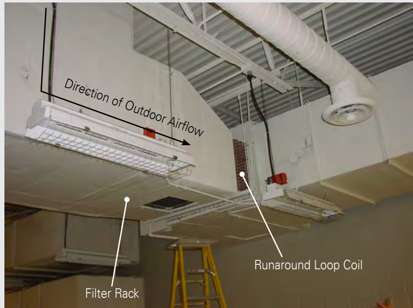
Figure 1.5-D Outdoor Air Portion of Runaround Energy Recovery Ventilation System
