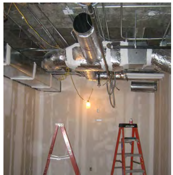
Figure 1.4-G Two Teams of Installers Working at the Same Construction Site: One Team Covered and Protected the Ductwork and the Other Did Not Photographs courtesy of Wayne Thomann.
