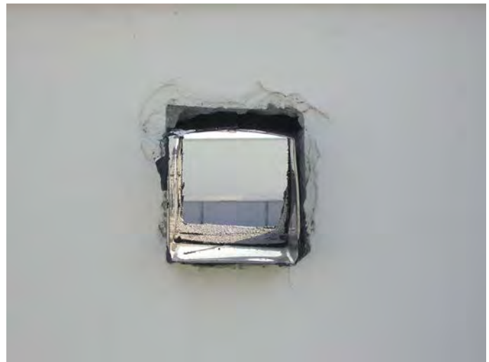
Figure 2.1-O Scupper without Sealant or Flashing Photograph copyright Liberty Building Forensics Group®.
