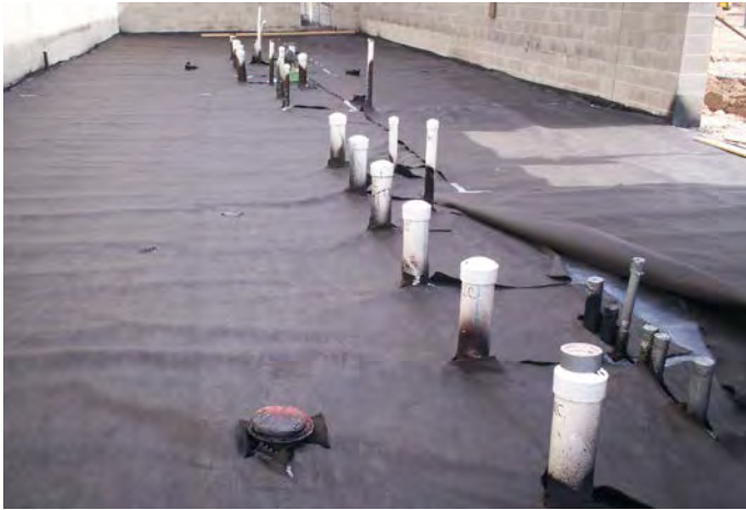
Figure 3.4-F Protective Layer Laid Over Solidified Spray-Applied Membrane Photograph copyright CETCO.
