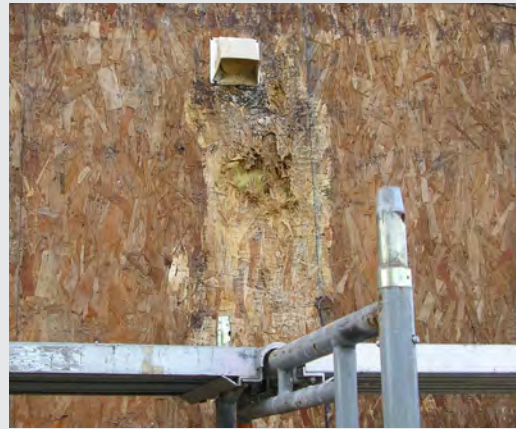
Figure 2.1-C Damage from Failure at Vent Penetration
