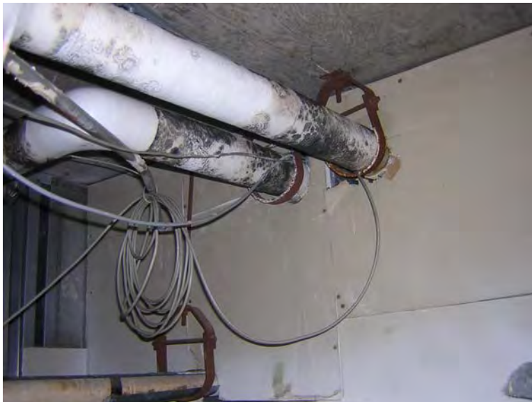
Figure 2.3-J Negatively Pressurized Return Air Plenum with Respect to the Outdoors Photograph courtesy of Wagdy Anis.
