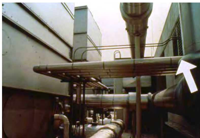
Figure 4.4-C HVAC Inlet Located within 13 ft (4 m) of a Double-Cell Cooling Tower Photograph courtesy of Phil Morey.
