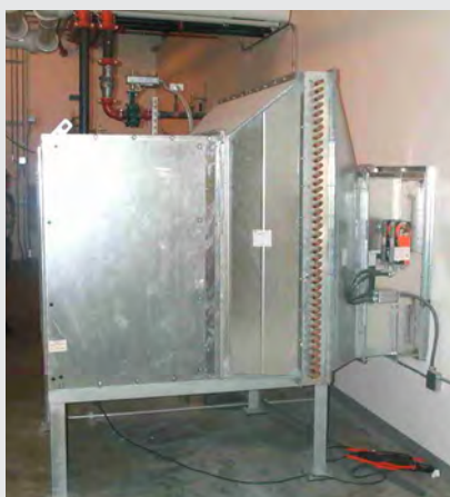
Figure 7.2-C Close-Up of Minimum Outdoor Air Intake Fan
