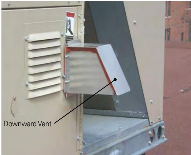
Figure 3.2-F Downward-Facing Vent Photograph copyright Battelle Memorial Institute.
