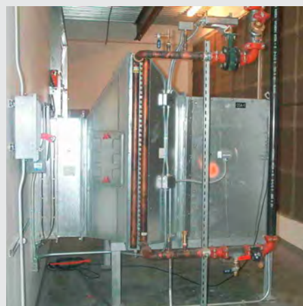
Figure 7.2-D Close-Up of Main Air Filters
