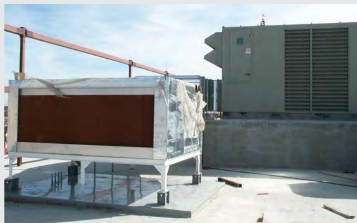
Figure 3.2-O Indirect Evaporative Cooler
