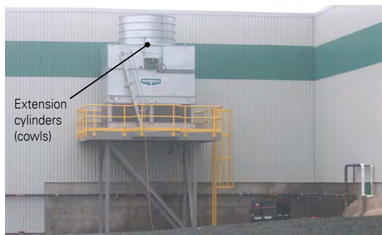
Figure 3.2-C Cooling Tower with Too Few Extension Cylinders (Cowls) Added to the Exhaust Plume Photograph copyright Evapco, Inc.
