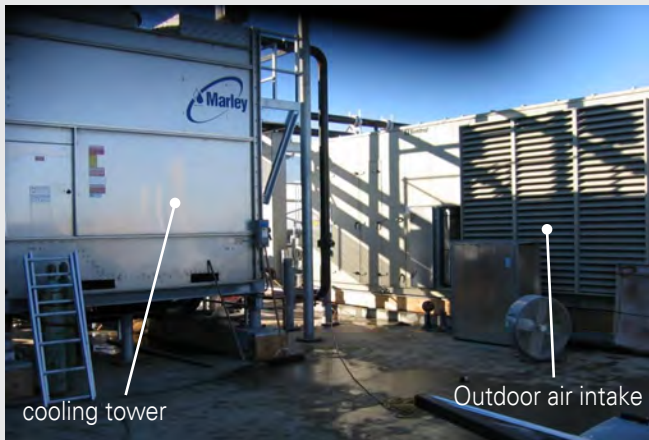
Figure 3.2-J Cooling Tower Located Near Outdoor Air Intake
