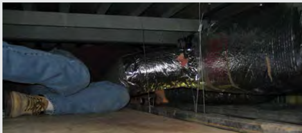
Figure 4.3-C System Location Limits Access
