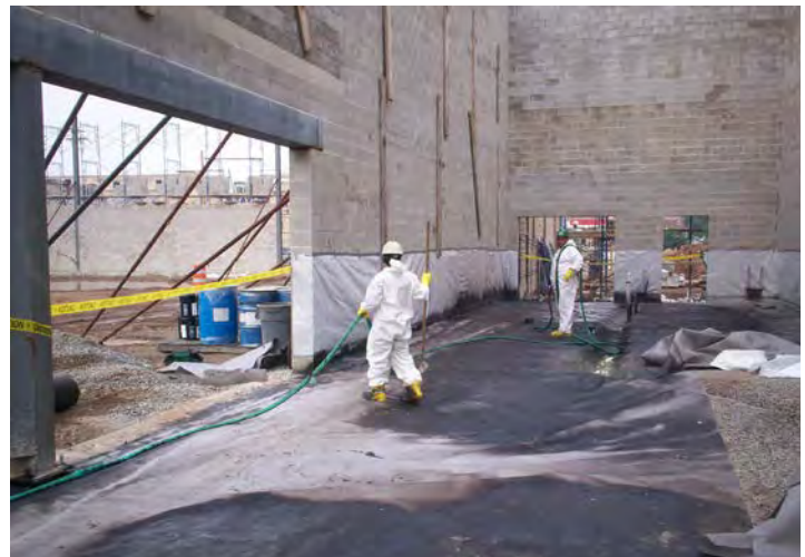
Figure 3.4-E Gas Vapor Barrier Membrane Being Sprayed on Base Fabric Photograph copyright CETCO.
