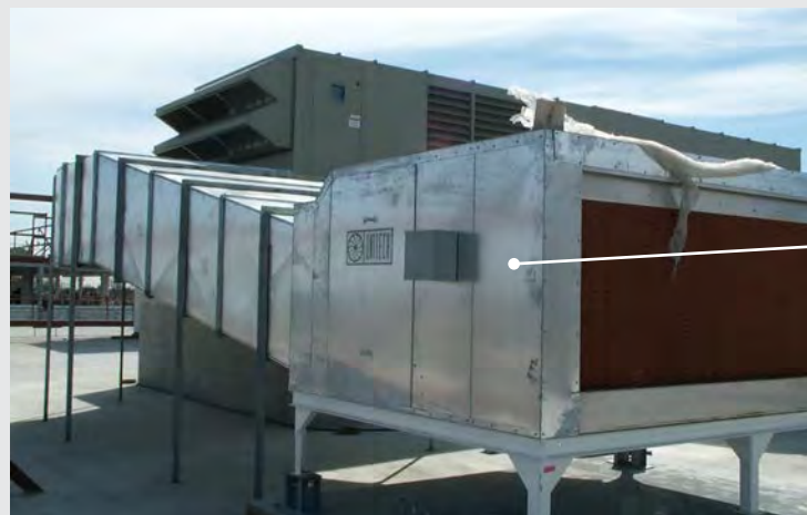
Figure 3.2-N Relocated Outdoor Air Intake
