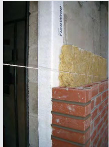
Figure 3.6-B Exterior Wall of Parged CMU
