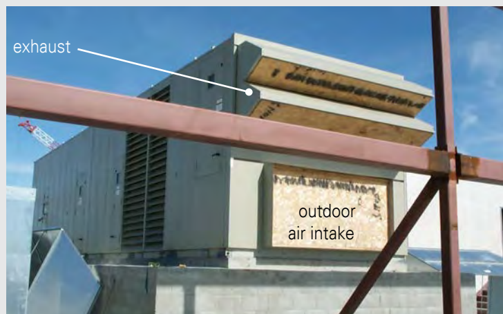
Figure 3.2-M Packaged HVAC Unit
