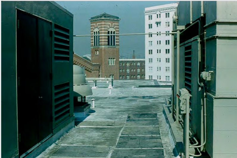
Figure 6.3-B Relative Location of Exhaust Fan to Intake Louvers
