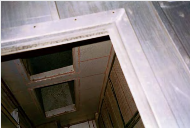
Figure 7.5-I Eroded Gasketing on Filter Access Door
