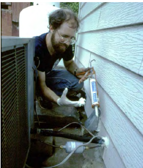
Figure 3.6-D Sealing a Potential Pest Entry Route around the Refrigerant Lines for an Air Conditioner Photograph courtesy of Terry Brennan.
