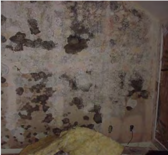
Figure 2.3-1 Humid Outside Conditions and Design Errors Combine to Cause Severe Mold Problems at a Luxury Hotel Photograph copyright CH2M HILL.
