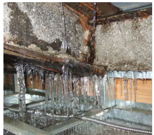
Figure 2.1-Y Ice Dam Failure Photograph copyright Liberty Building Forensics Group®.
