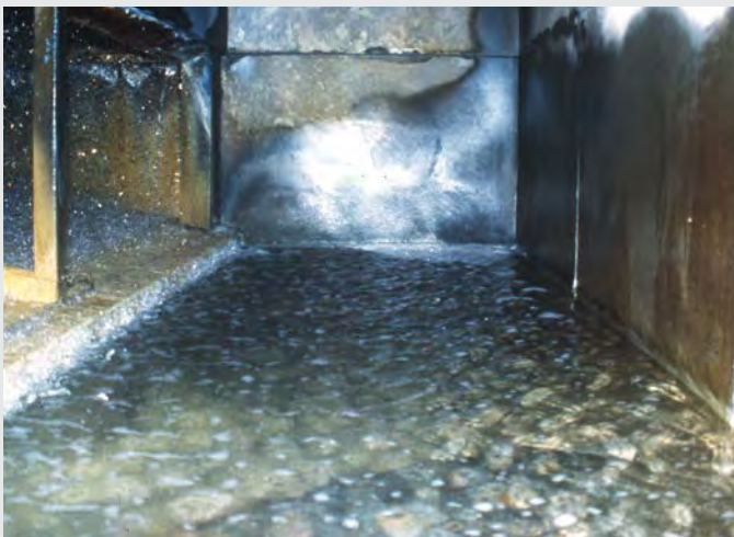
Figure 4.4-D Relatively Clear Water in the Basin of the Cooling Tower on the Roof of Building B Photograph copyright Janet Stout, Special Pathogens Laboratory.
