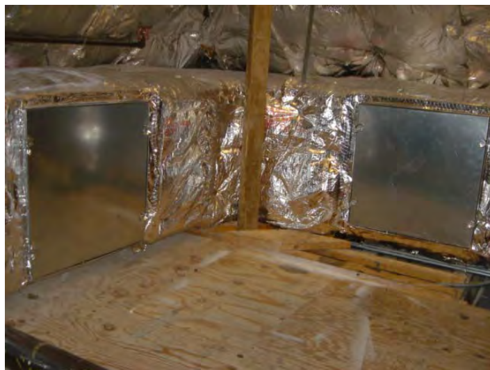
Figure 4.3-L Multiple Reusable Access Panels Installed at a Supply Duct Photograph courtesy of Wayne Thomann.
