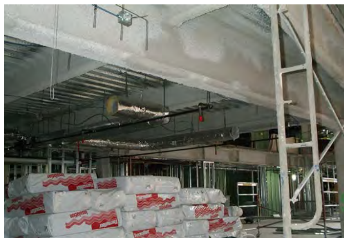
Figure 5.1-M Insulated Surfaces: Wrapped HVAC Ducting, Structural Member Spray-On Insulation Photograph courtesy of Leon Alevantis.
