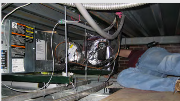
Figure 4.3-D All System Components not Readily Accessible
