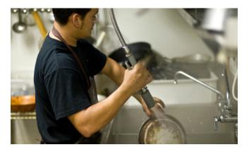
per year, equivalent to the amount of water needed to wash nearly 4,800 racks of dishes. Because kitchens use hot water to rinse dishes, installing a highefficiency PRSV can reduce a commercial kitchen's annual natural gas use by more than 5,700 cubic feet per year. That's enough energy to run its convection oven 12 hours per day for three weeks.
