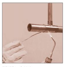
FIGURE 25: Soldering
