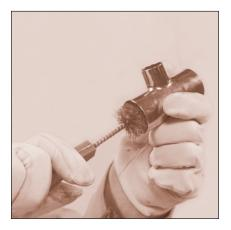
FIGURE 17: Cleaning: Fitting Brush
