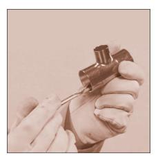
FIGURE 19: Fluxing: Fitting
