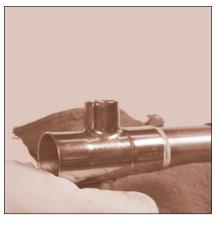
FIGURE 21: Removing Excess Flux
