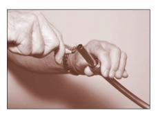
FIGURE 30: Reaming Prior to Flaring the Tube End
