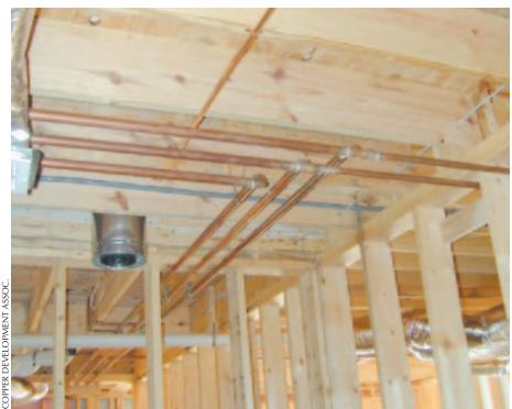
**Figure 5.** In this home, <sup>3</sup>/4-inch copper lines tee off from the 1-inch mains on the left.
