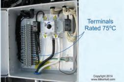
Conductors terminating on equipment rated 75°C are sized in accordance with the ampacities listed in the 75°C temperature column of Table 310.15(B)(16), provided the conductors have an insulation rating of at least 75°C.
