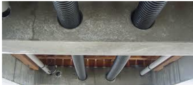
Figure 79: Water Service pipe installation
