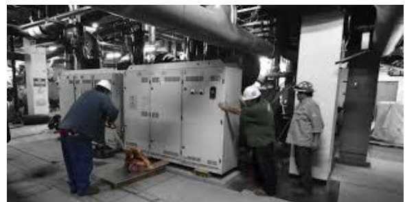
Figure 185: Securing to foundation
