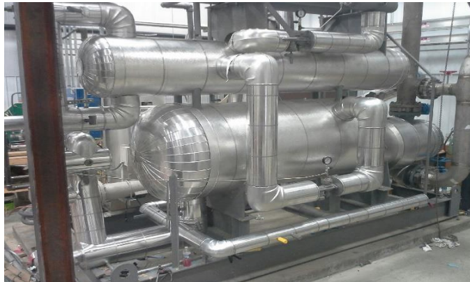
Figure 171: chilled water insulation
