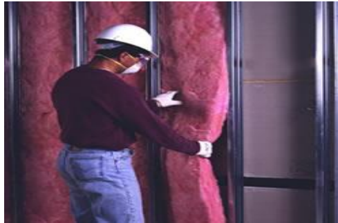
Figure 140: Acoustic lining
