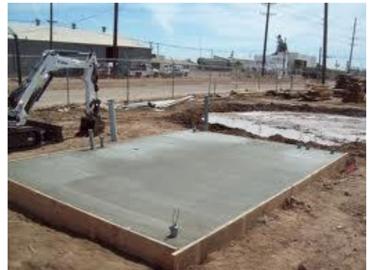
Figure 122: Generator foundation
