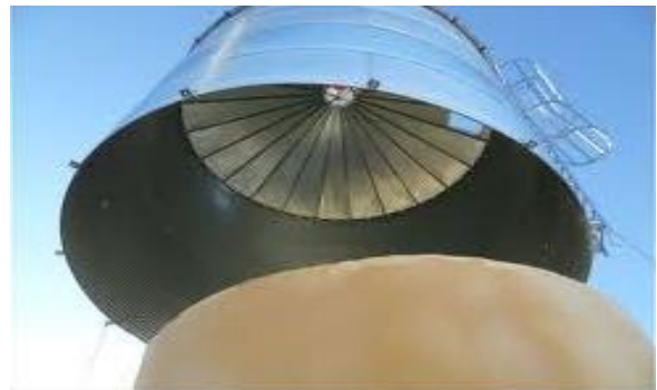
Figure 64: shell, roof and stair installation
