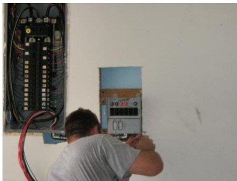
Figure 198: transfer switch
