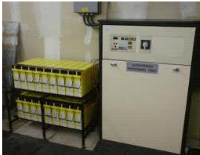
Figure 202: Central battery system
