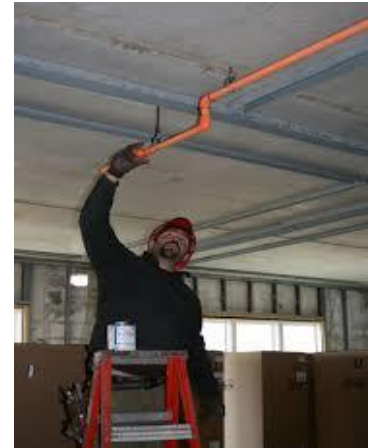
Figure 44: Sprinkler Pipework
