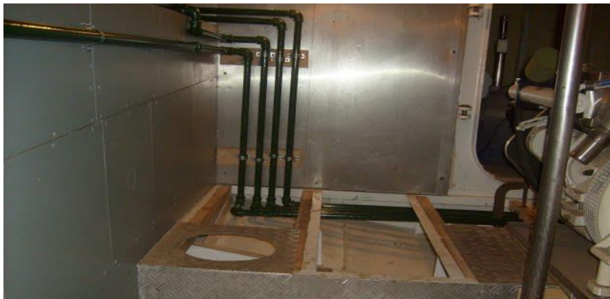
Figure 126: Fuel piping
