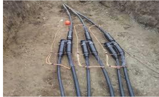
Figure 195: Cable splicing
