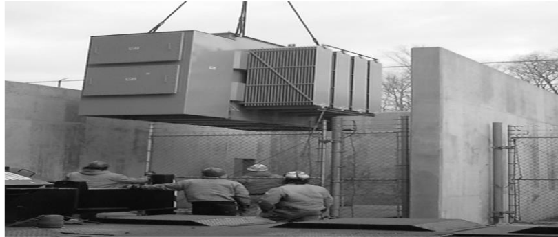
Figure 186: transformer installation
