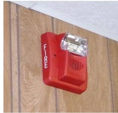
Figure 238: Notification appliance
