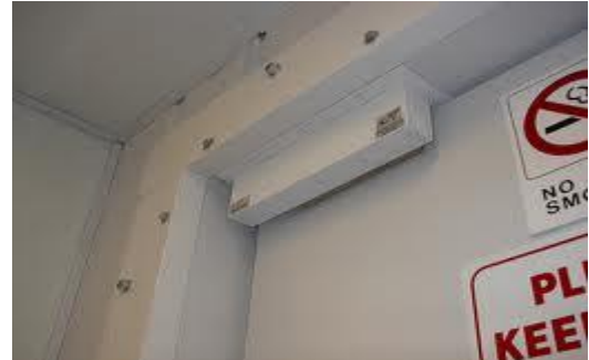
Figure 231: Magnetic lock
