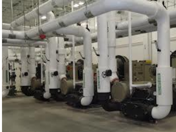
Figure 127: HVAC piping and pumps
