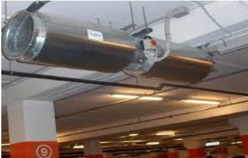
Figure 165: parking supply fan
