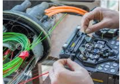
Figure 213: Splicing
