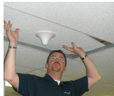
Figure 220: In-building antenna installation
