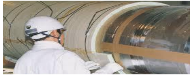
Figure 131: insulation material installation and securing
