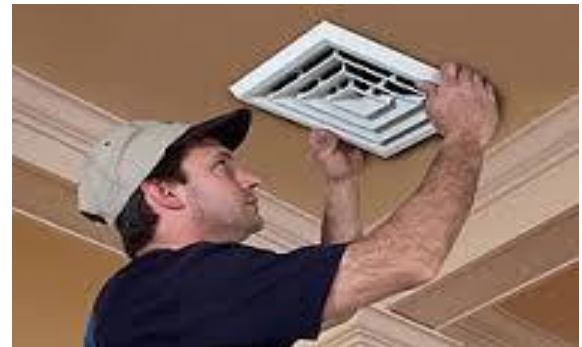
Figure 147: Diffuser installation
