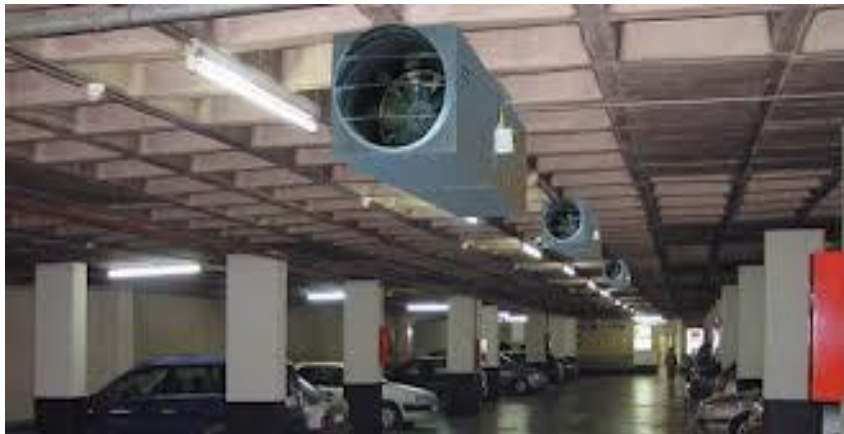
Figure 164: parking exhaust fan
