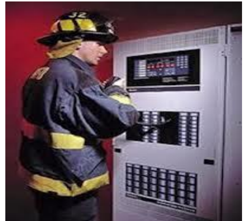
Figure 239: Fire alarm control units
