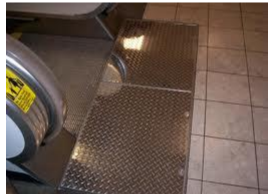
Figure 33: Landing Plate
