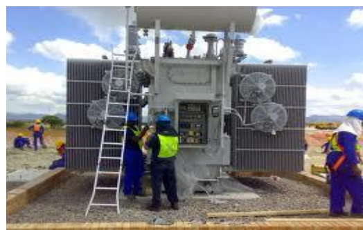
Figure 188: transformer site assembly
