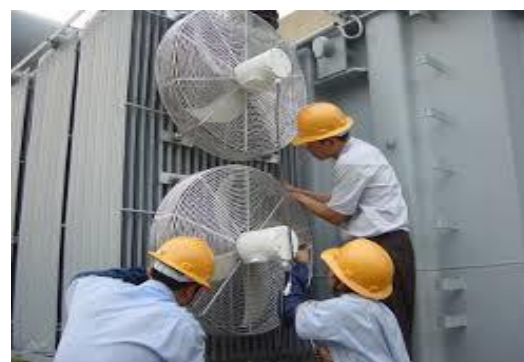
Figure 189: Cooling fans installation
