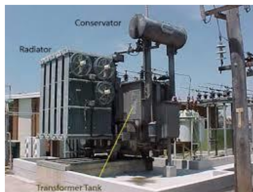
Figure 190: Conservator installation
