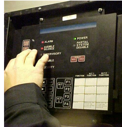
Figure 240: Remote on-site annunciation
