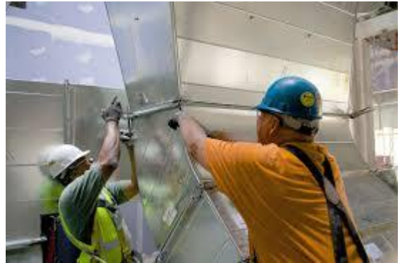
Figure 138: Duct installation
