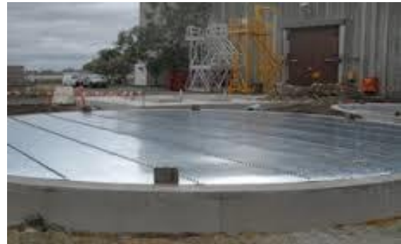
Figure 63: Tank support/foundation
