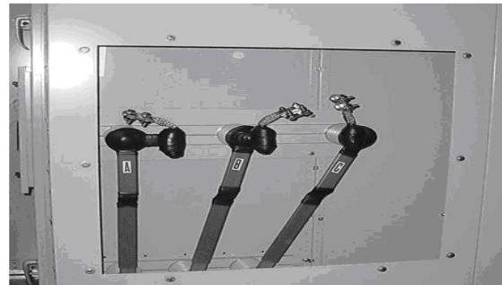
Figure 182: Connection to transformer
