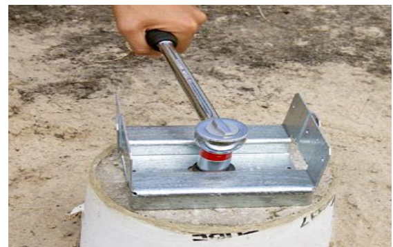
Figure 156: anchor bolt tightening
