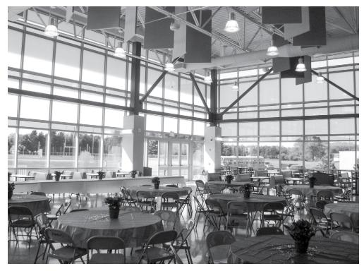
**Figure 6.** Frosted glass above, clear glazing below. The area below the frosted glazing is acceptable vision glazing. This space also has multiple views more than 90 degrees apart. Photo by Todd Reed.
