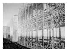
**Figure 4.** Fritted glass with horizontal strips of clear glazing. The area between the upper and lower portions of fritted glass is acceptable vision glazing. Photo by Michael Spillers.
