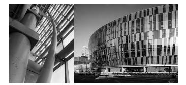
**Figure 5.** Fritted glass with vertical panels of clear glazing. The glazing between the fritted panels is acceptable vision glazing. Photo by Michael Spillers.
